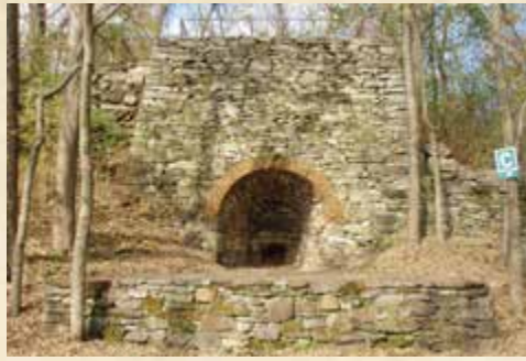
Lime kilns were loaded with limestone rocks and fuel. The resulting heat transformed the stone into lime powder which was then spread on the fields.
